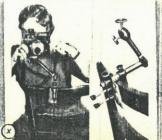
Microp totography demands that the camera be supported firmly, at the categot height above the microscope tube. The most suitable stand has two feet at right angles to each other (using 1½ leg sections each), providing a secure support for the assembly around the centre of gravity. The complete formula is:
